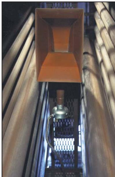
*Figure 6 - Acoustic cleaner installed*
