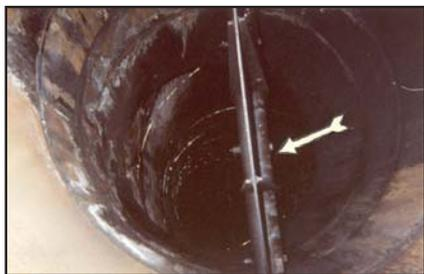
Figure 9 - Corroded Dividing Plate
