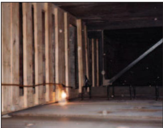
Figure 7: Final design flow distribution baffles
