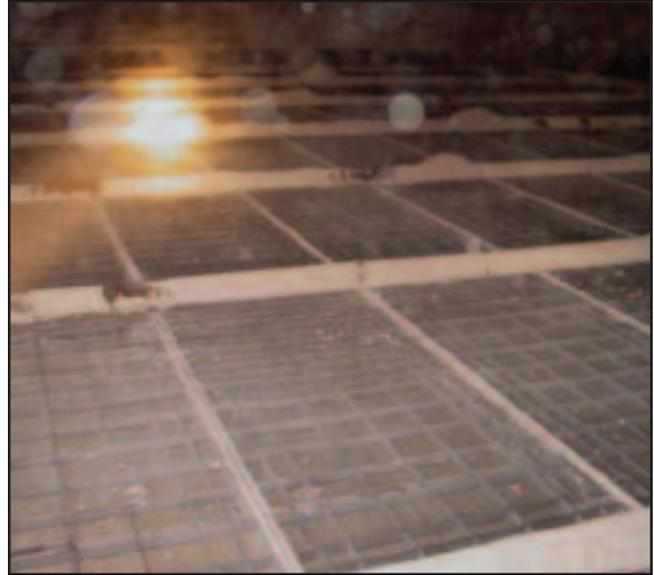
Figure 3: A View Inside a SCR Reactor that is being cleaned solely by acoustic cleaners.
