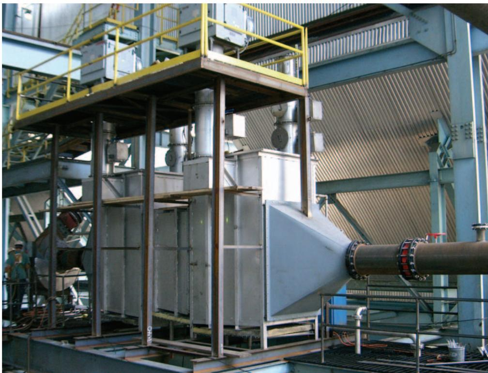
Figure 3: Hybrid Dry-Wet ESP™
