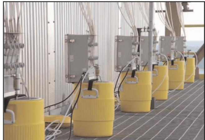
Figure 6: Multi-point Automated Sampling System (MASS)
