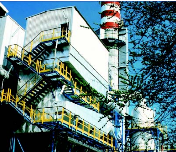
Municipal Solid Waste Incineration 16 MW – 65,000 ACFM
