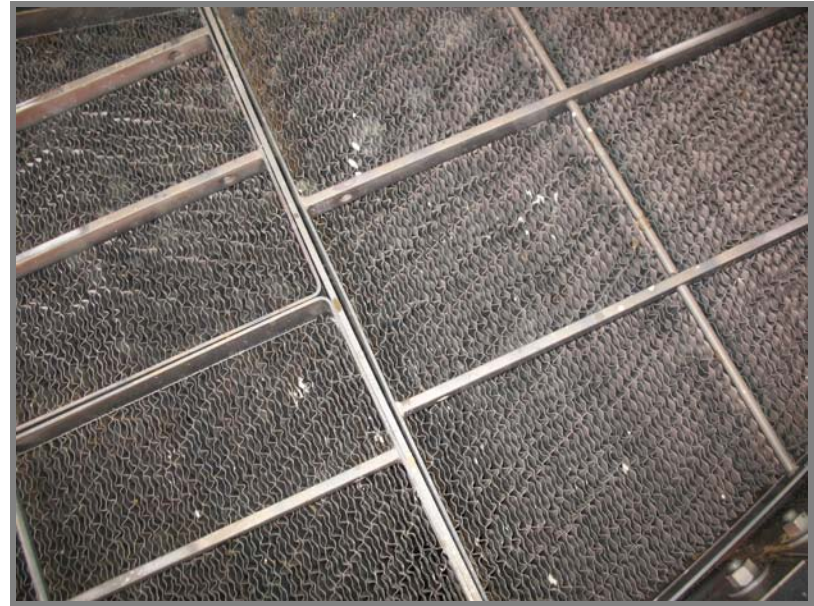
APH after 8 week trial of PreAPH hydrate injection
